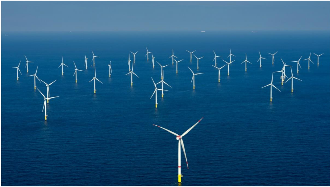
Figure 2.6 Vineyard Wind 1 wind farm layout (POWER TECHNOLOGY, 2021)
